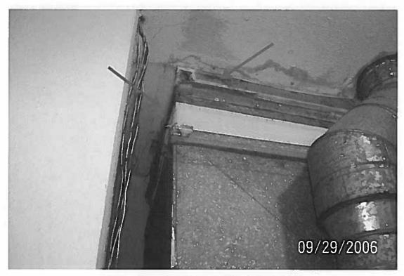
2504 - Asbestos HVAC Tape & Vibration Boot - Note mold growth and water damage from condensation
