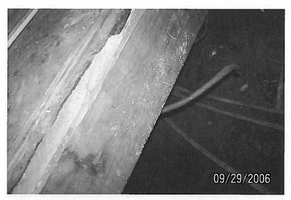
2504 - Mold & Mildew growth on floor joist at hatch
