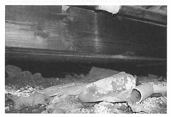
2510 - Views under the floor - note mold growth on debris under the floor
